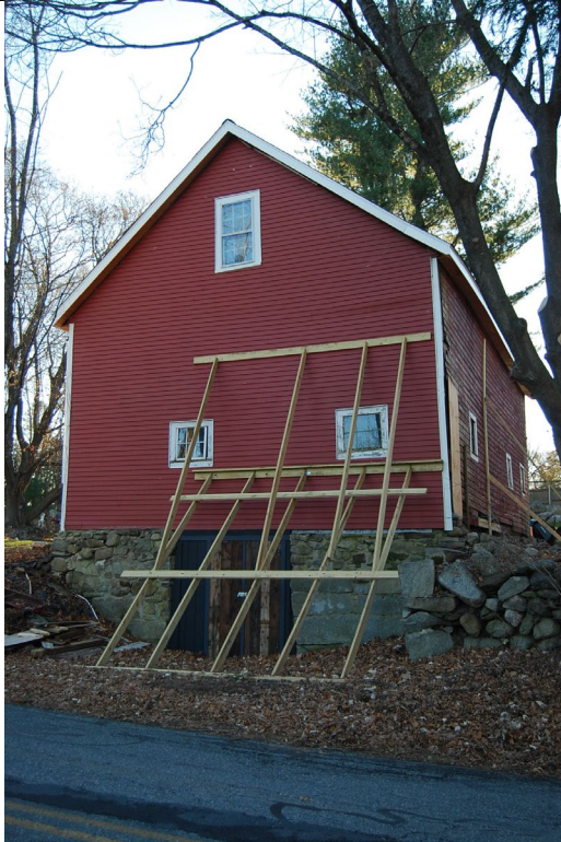
Barn. View looking west at northeast elevation.
