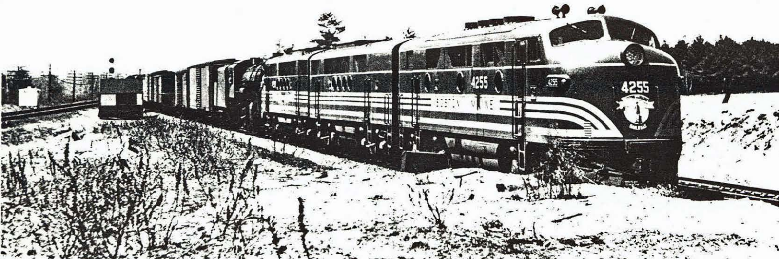
A Worcester to Portland freight negotiates the new cut-off trackage which branched off the Fitchburg main at Willows. An A-B-A diesel lash-up is leading a K-8 2-8-0 in this photo by Dana D. Goodwin taken on May 11, 1947. In the scene below we find RS-3 no. 1539 on Train 805 to Lowell pulling into the station at Graniteville during the last week of local passenger service, April 22, 1953.
