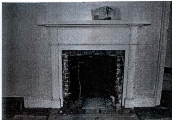
1st floor North (right) room
