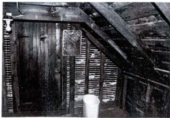
Facing main house
