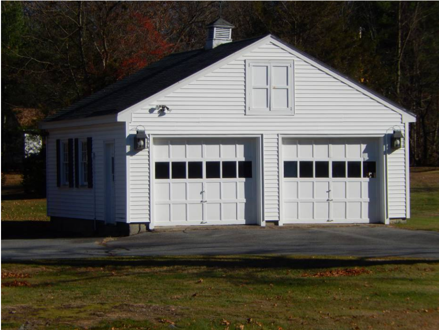
Garage, facing northeast. November 2015.
