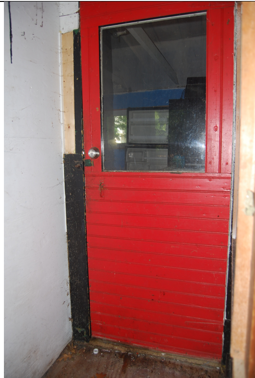
Detail. Recessed entrance at northeast corner of house.
