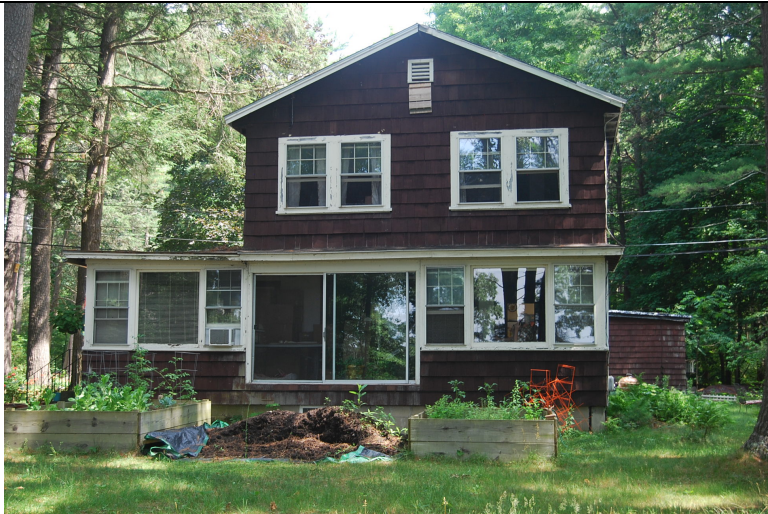
View looking northeast. South elevation.
