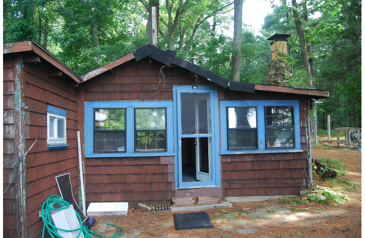
Photo 1. View looking northeast. Façade (south) elevation of main block. Corner ell at left.
