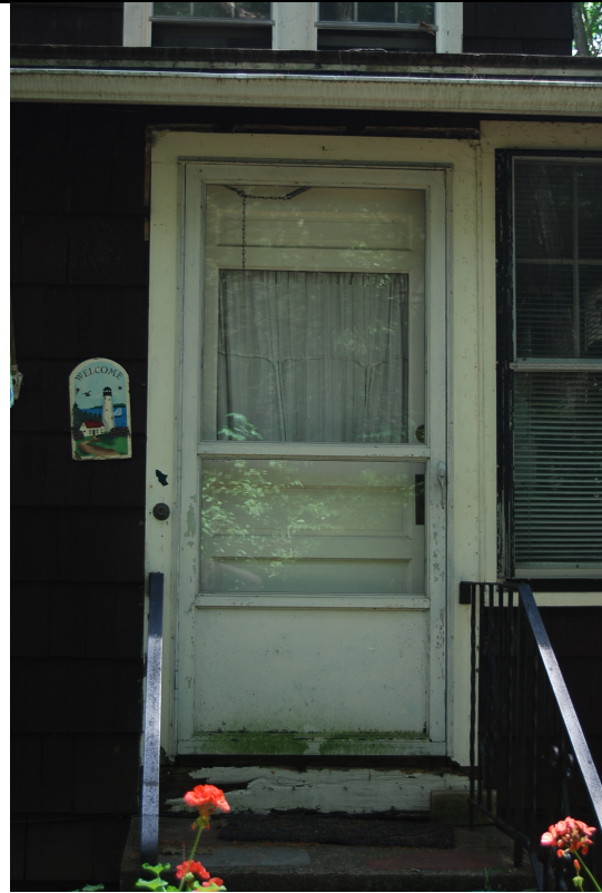
Detail. Entrance. West façade.
