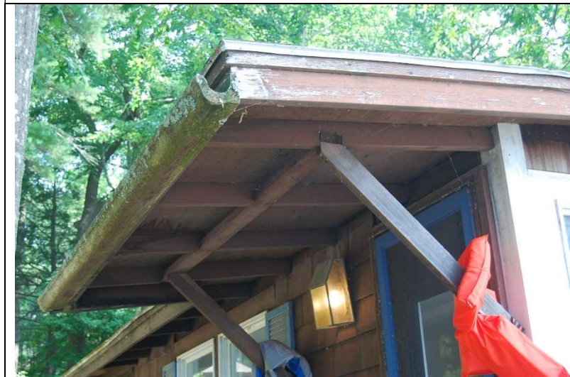
Detail. Wood gutter.
