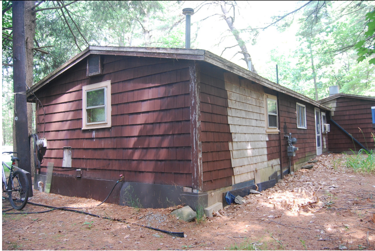
View looking north. South and east elevations of main block.
