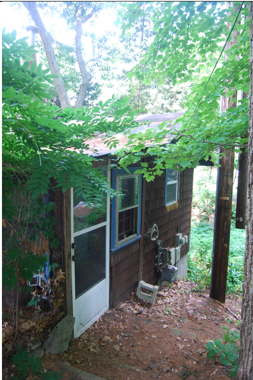
View looking west. North elevation.
