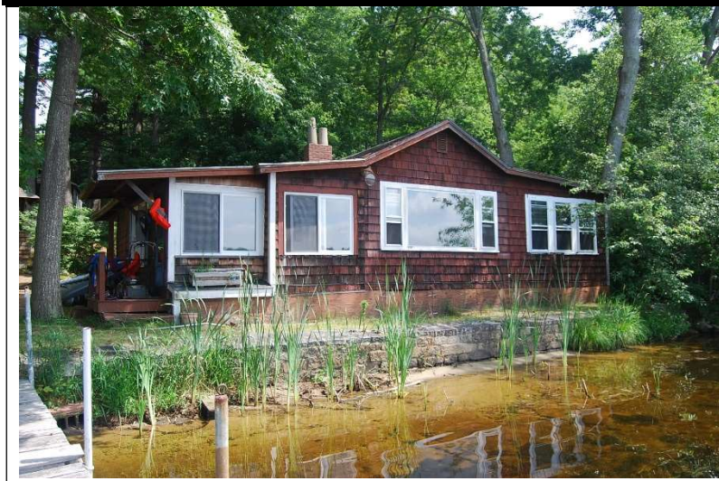
View looking northeast. South elevation.
