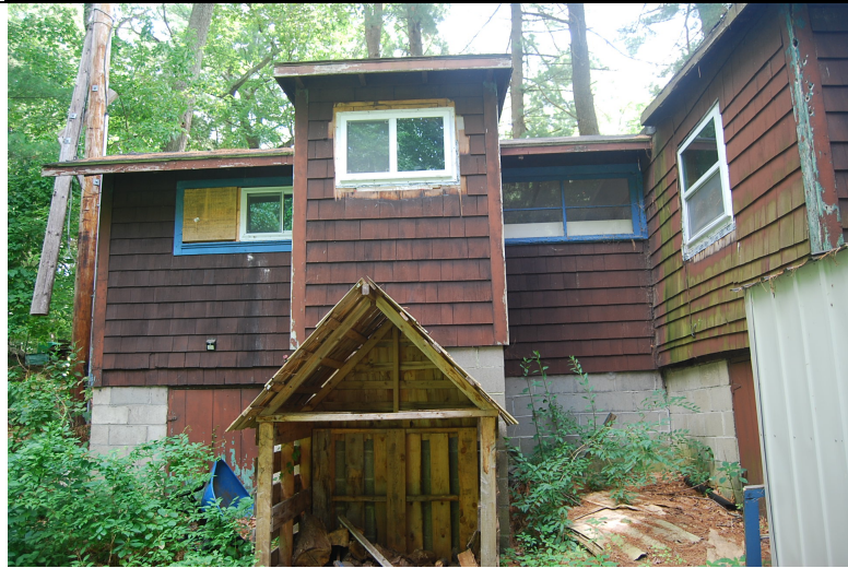
West elevation. View looking southeast.
