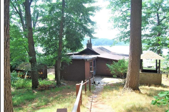
View looking south toward rear elevation of cottage and Hart Pond beyond. Well at right. Shed partially visible at left.
