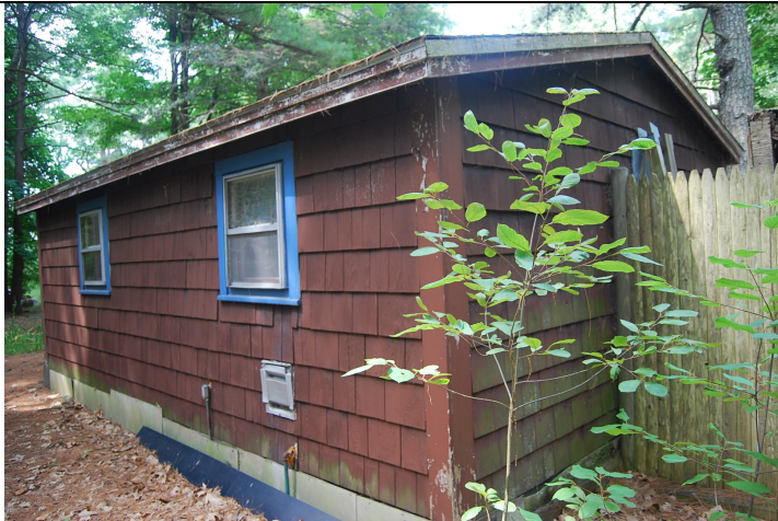
Ell. View looking southwest. East and north elevations
