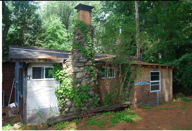
View looking northwest. East elevation.
