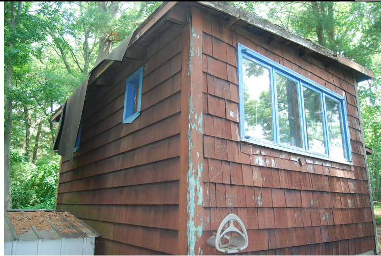
Corner ell at southwest corner of house. View looking east.
