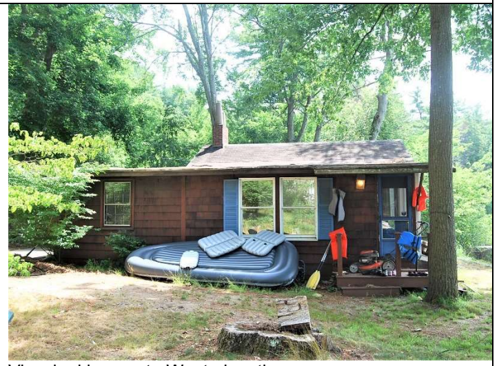
View looking east. West elevation.
