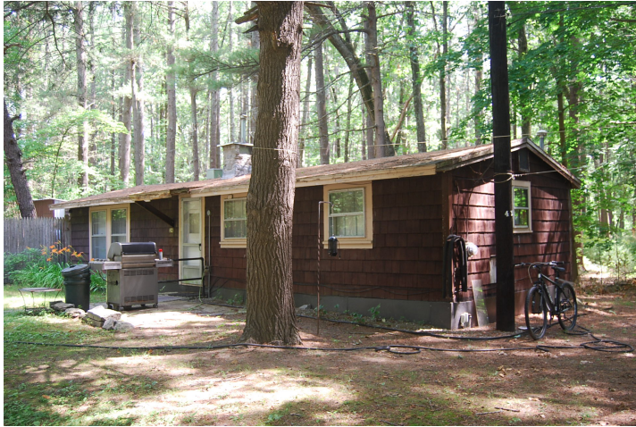
View looking northeast. Façade (west) and south elevations
