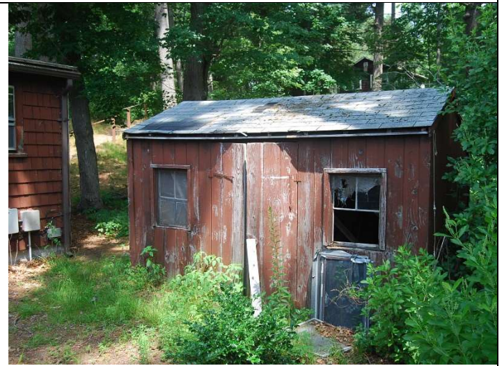
View looking north. Shed.
