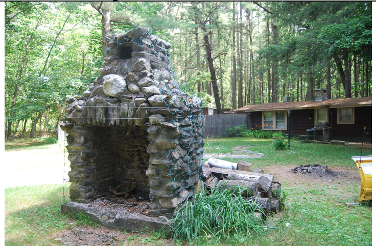
Fireplace. View looking northeast.
