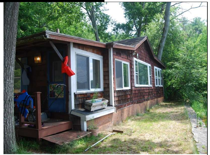
View looking east. West and south elevations.
