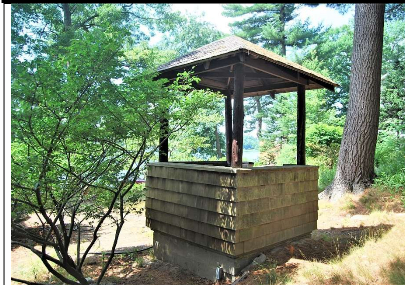
View looking southwest. Gazebo.
