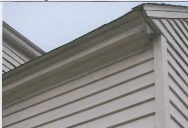
View looking southwest at remaining molded cornice.
