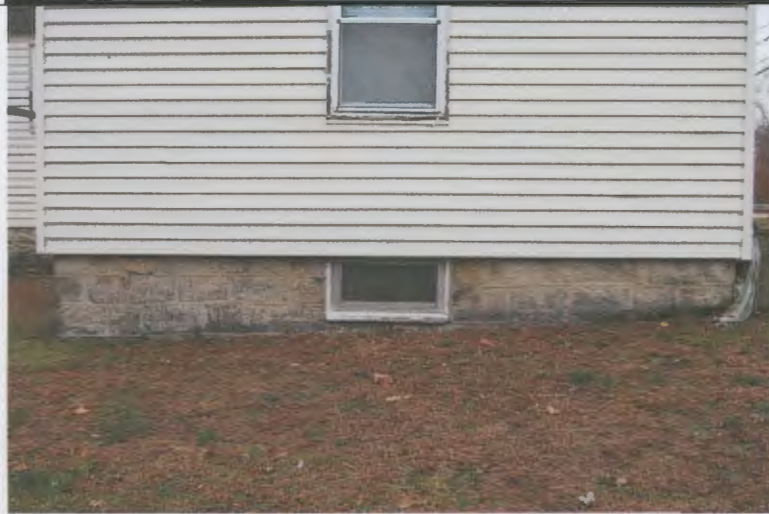
Masonry detail. South side elevation of main block.
