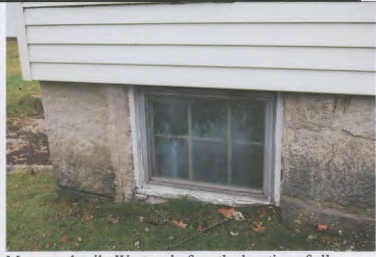
Masonry detail. West end of south elevation of ell.
