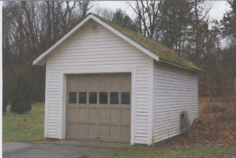
Garage. View looking south.
