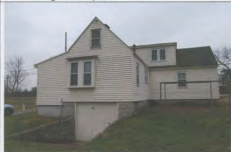
View looking east at rear elevation.
