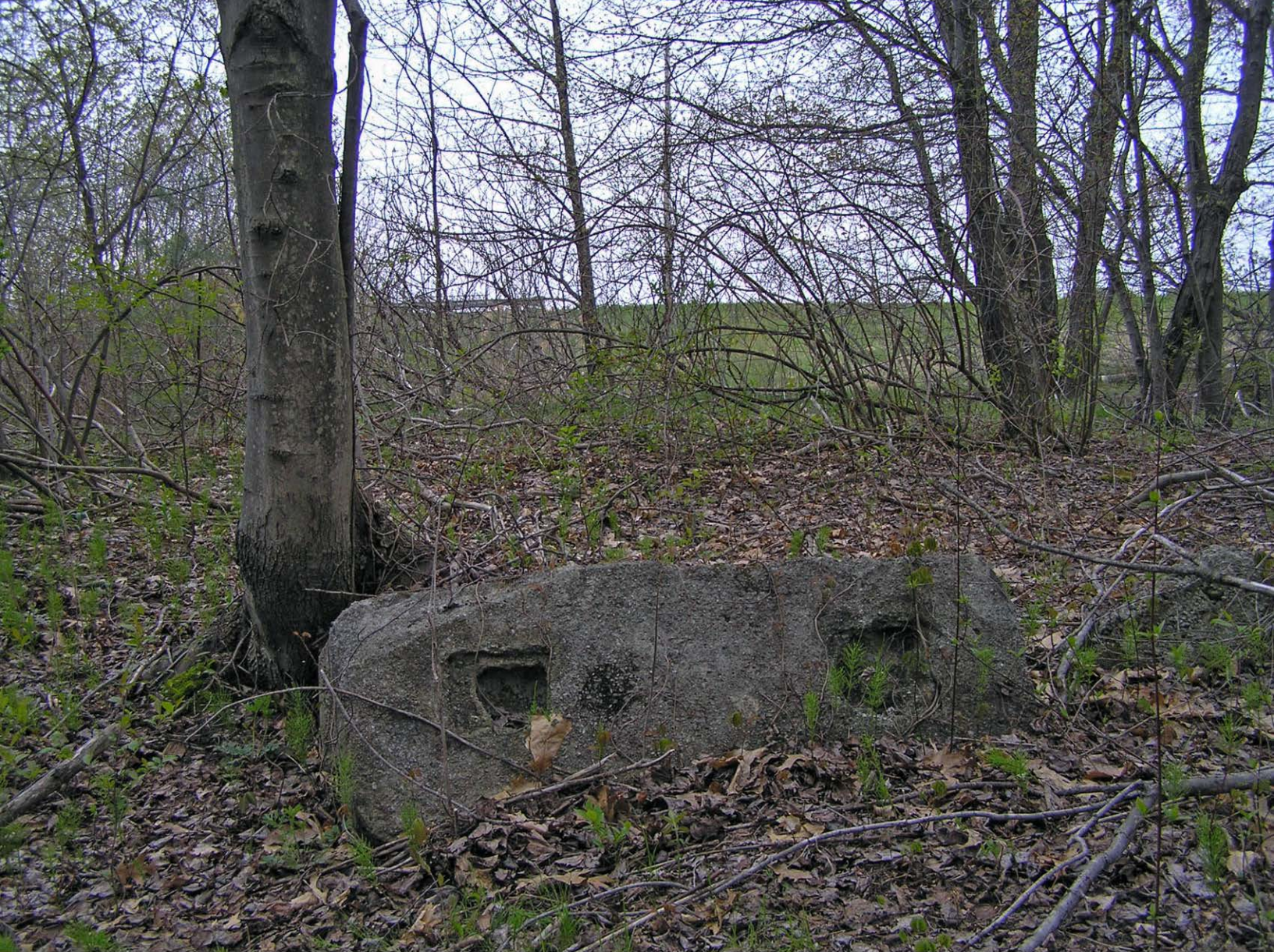
All that remains of the Boston Ice Co. storage buildings today is foundation blocks
