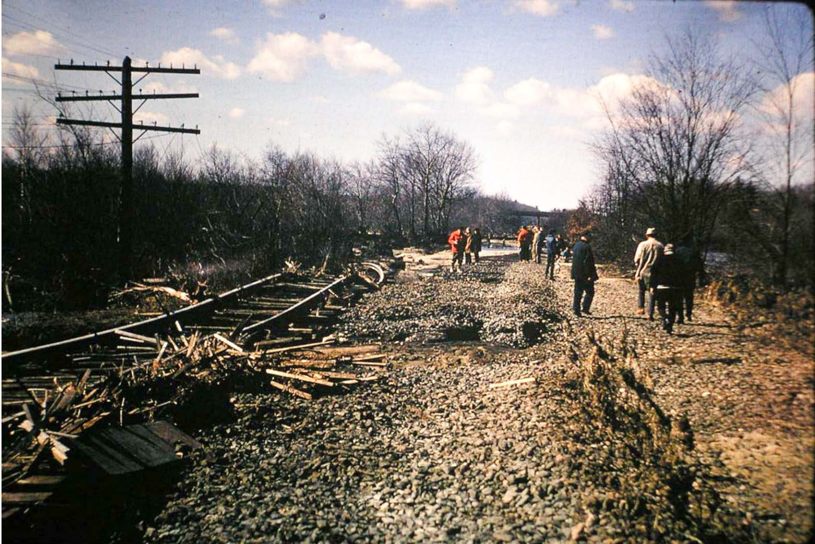
Stony Brook Railroad line looking toward Route 3 overpass
